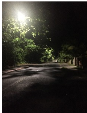
New LED lighting on Old Wokingham Road
